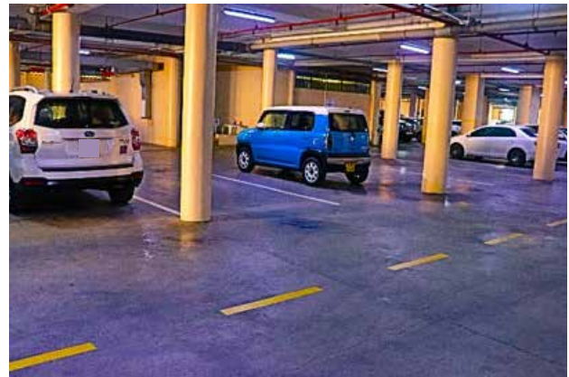
Basement parking area
